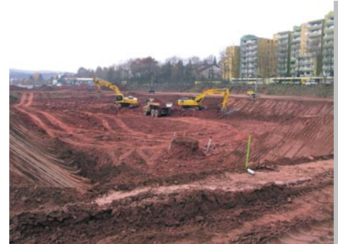
Heavy machinery digging up the red soil: excavation work started in 2003.
