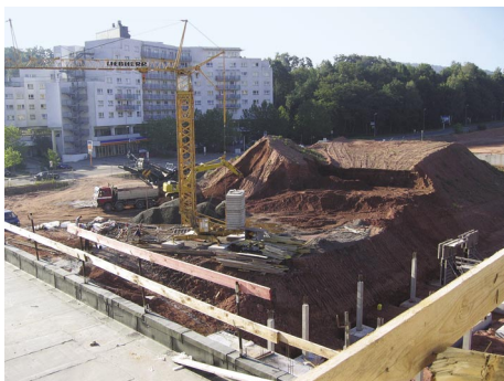
Approaching the finish line: By the end of the year 2005, the Day Care Center being built here will offer 30 slots.
